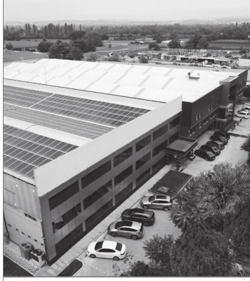
Yeşil Enerji We Care About Green Energy
